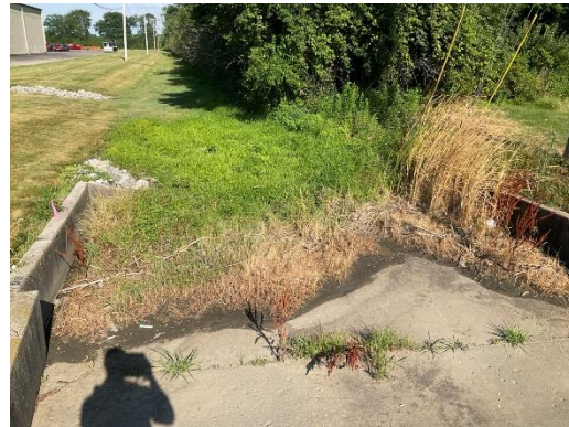
WOH-KLV-001 (PEM) Facing West (06/25/2024)
