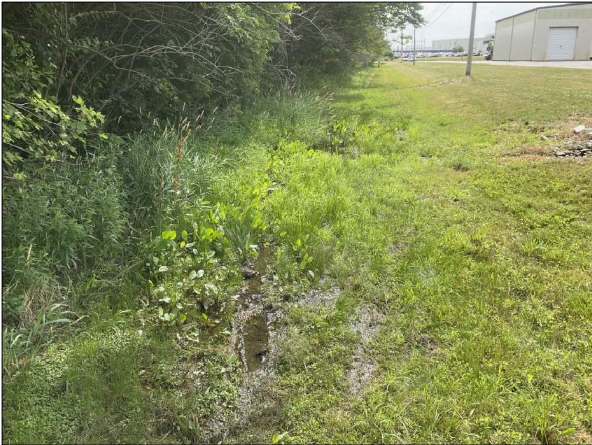
Photograph 1. General view of Project from near Structure 14006, facing east.
