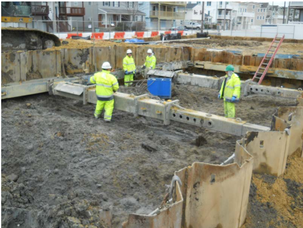
Installation of interior bracing
