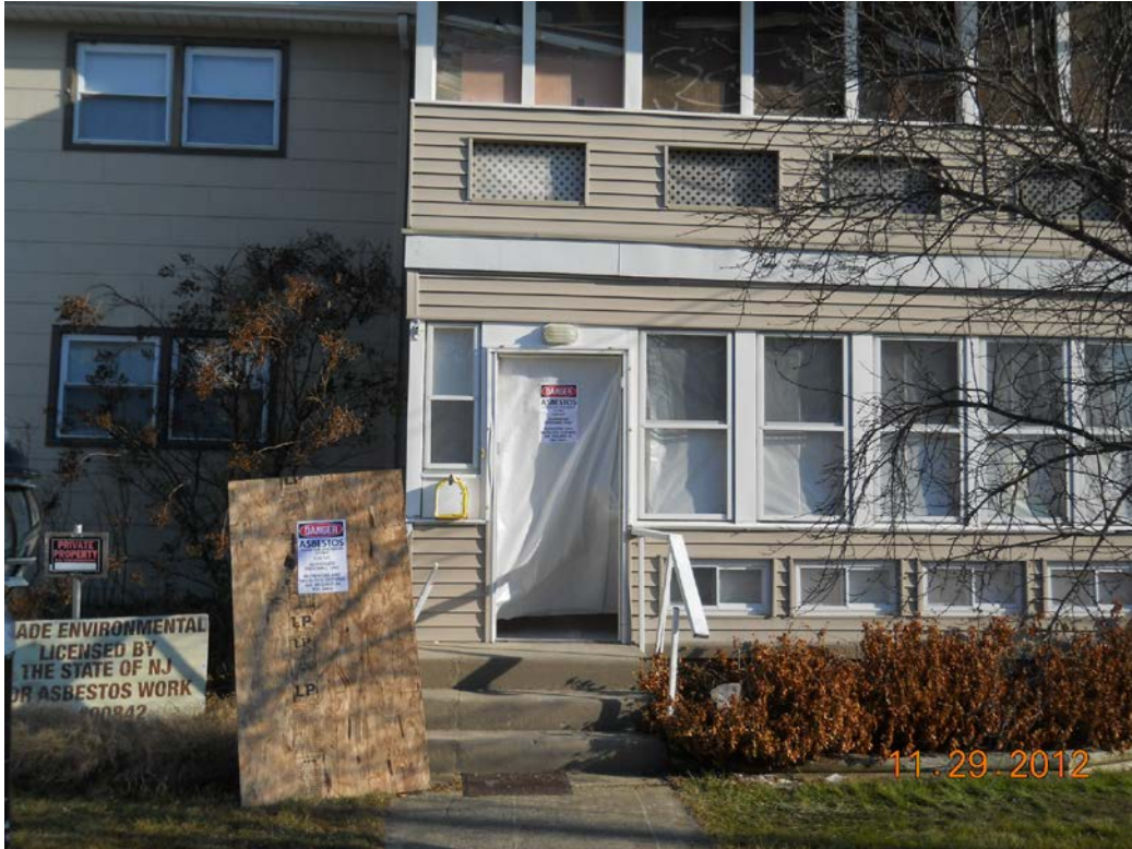
223 40 th Street asbestos abatement
