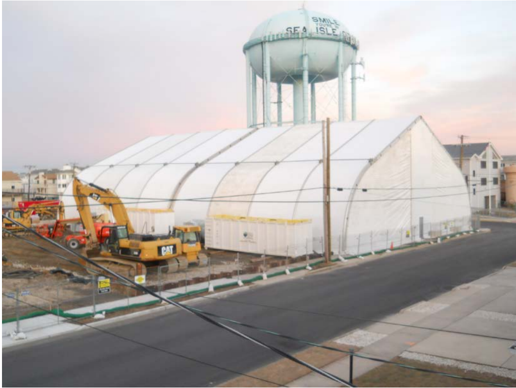
Temporary enclosure used during the Remediation Area 2 remedial action
