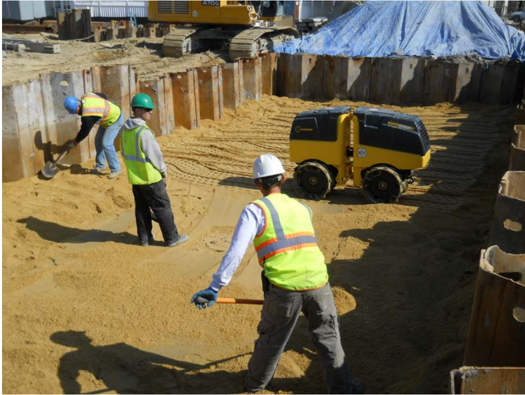
Backfilling and compacting excavation cell
