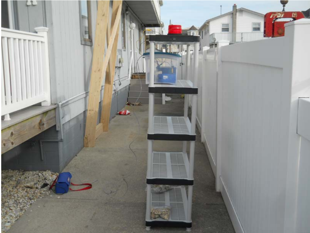
Vibration monitoring alarm system
