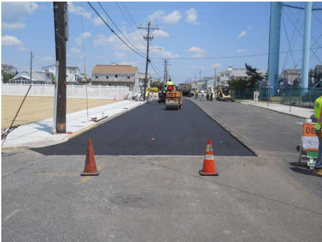
Repaving Central Avenue
