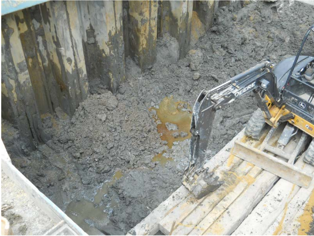
Product pooling in cell J2 during excavation
