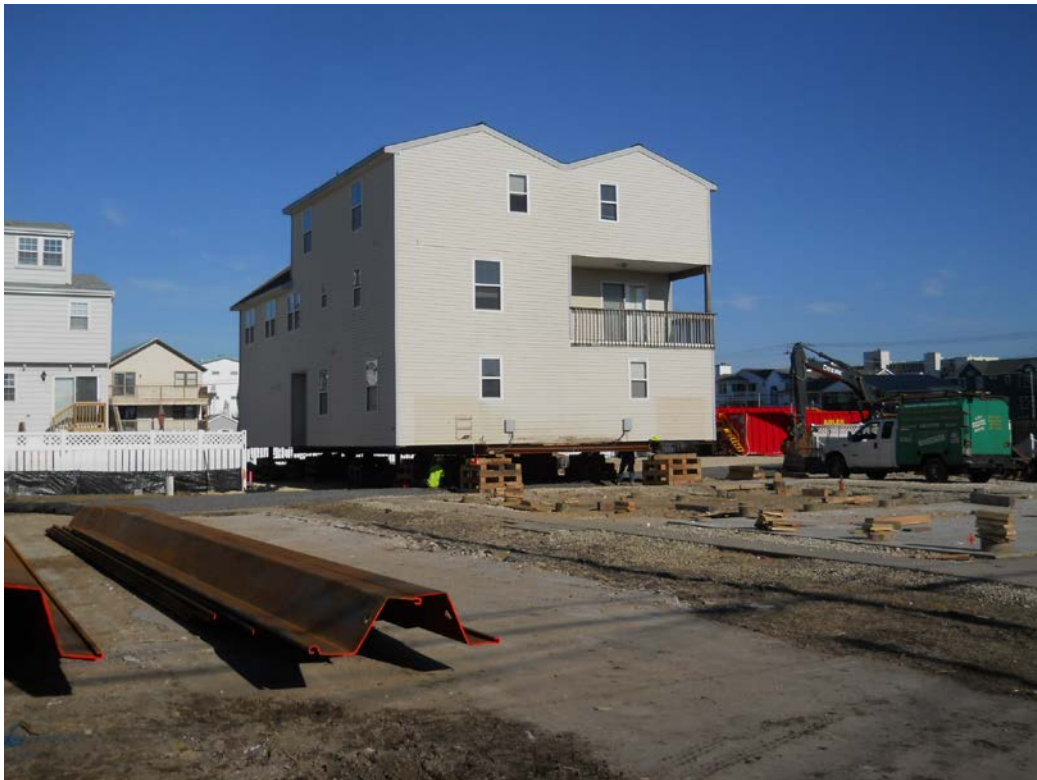
Relocating structure from 211 40 th Street to 214 39 th Street
