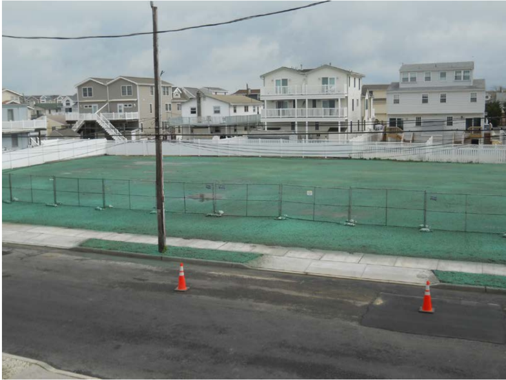
Remediation Area 1 after completion of site restoration
