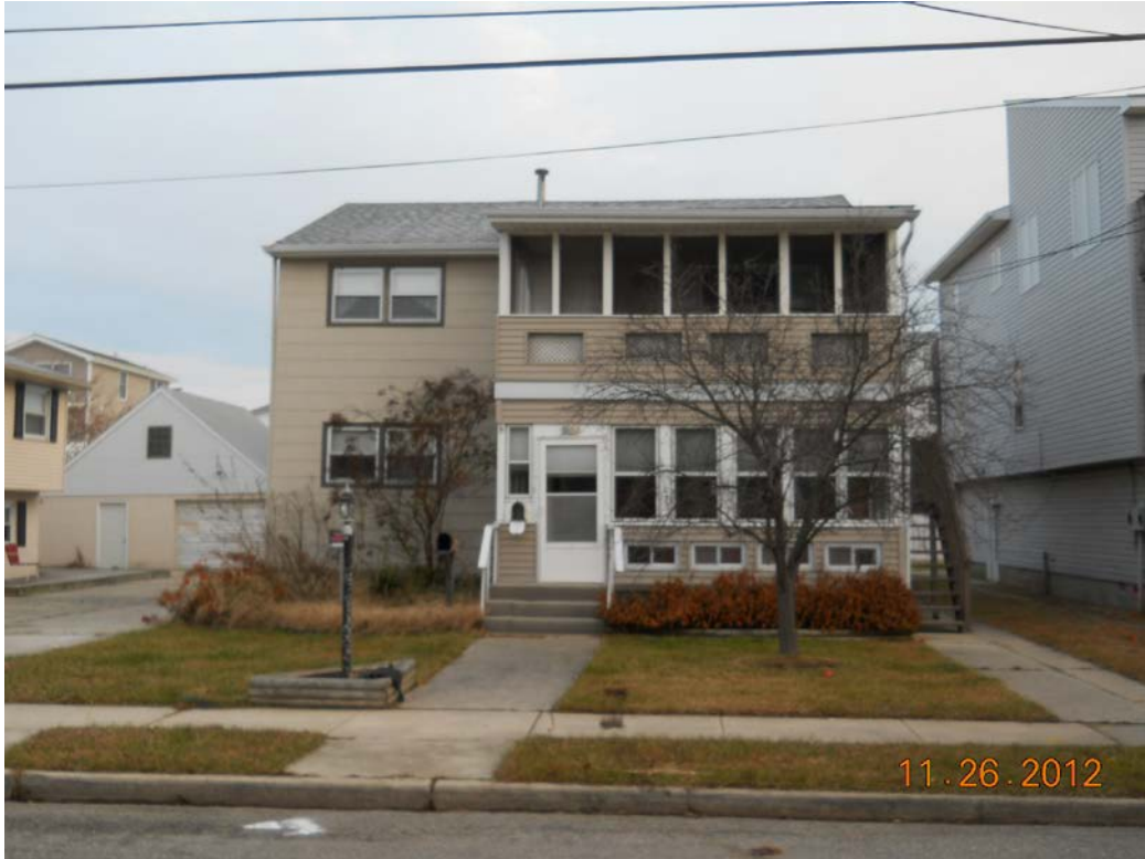
223 40 th Street prior to demolition
