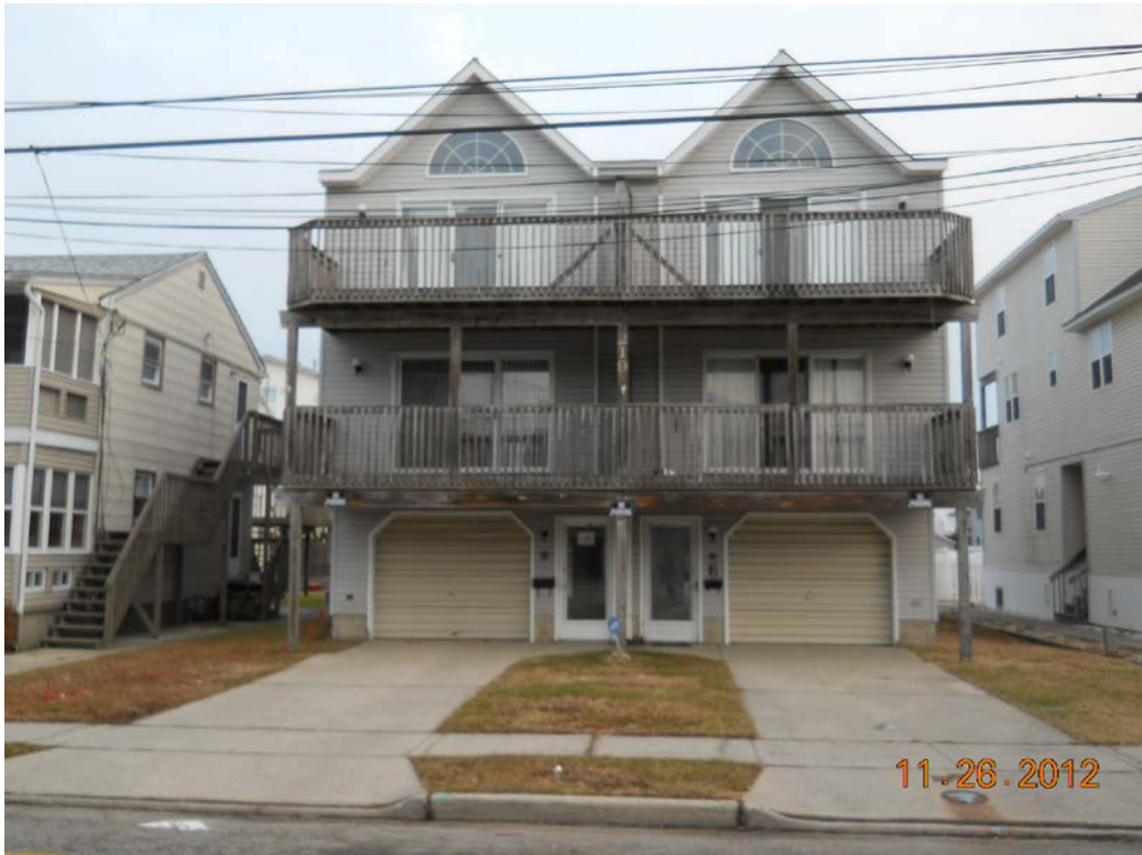
219 40 th Street prior to demolition
