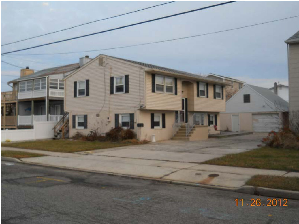
227 40 th Street prior to demolition
