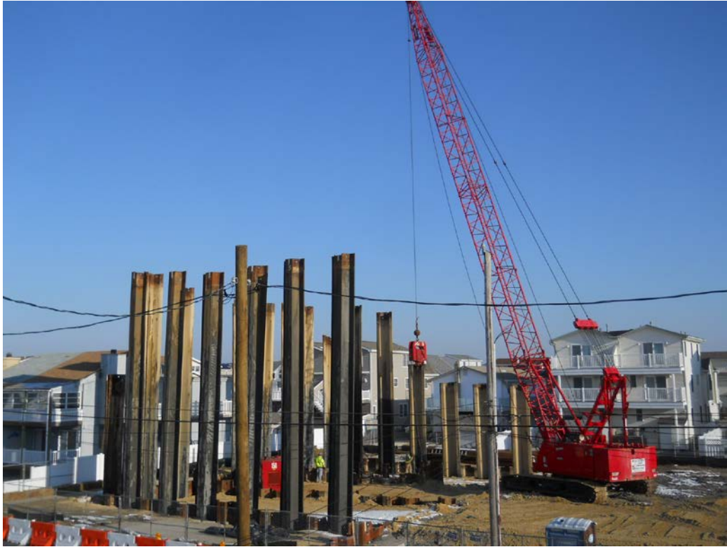
Sheeting installation for the Remediation Area 1 remedial action.
