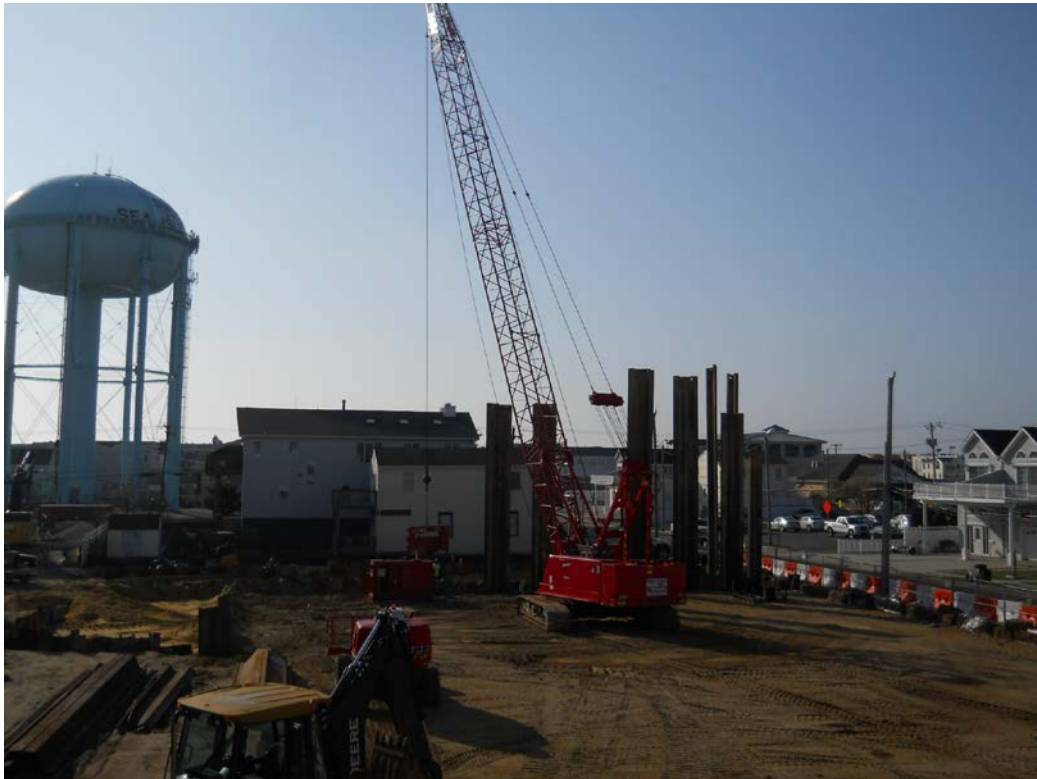
Sheeting removal at the conclusion of the Remediation Area 1 remedial action
