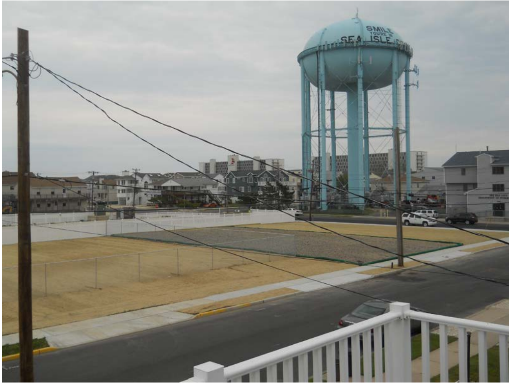
Remediation Area 2 after completion of site restoration
