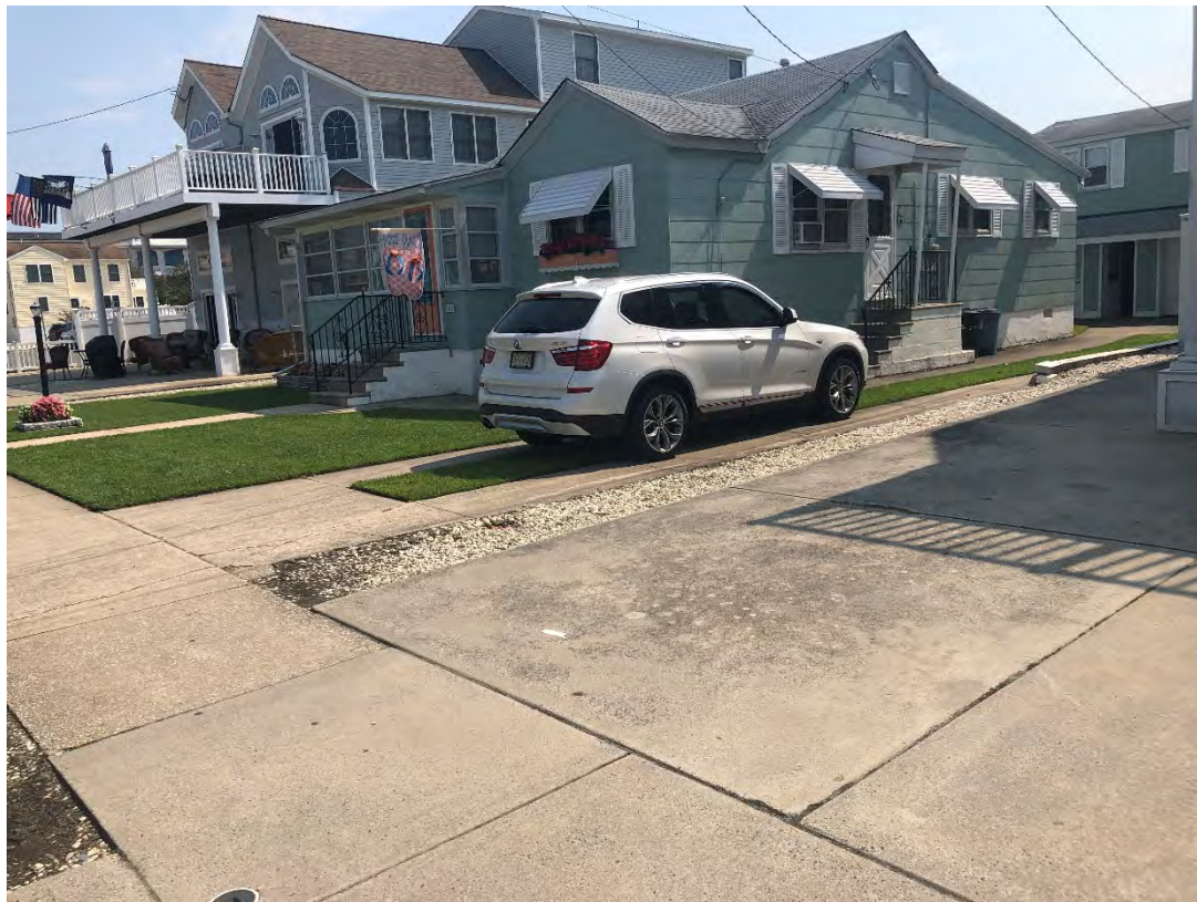
Photo No. 5 – West Front Exterior of 218 40 th Street
