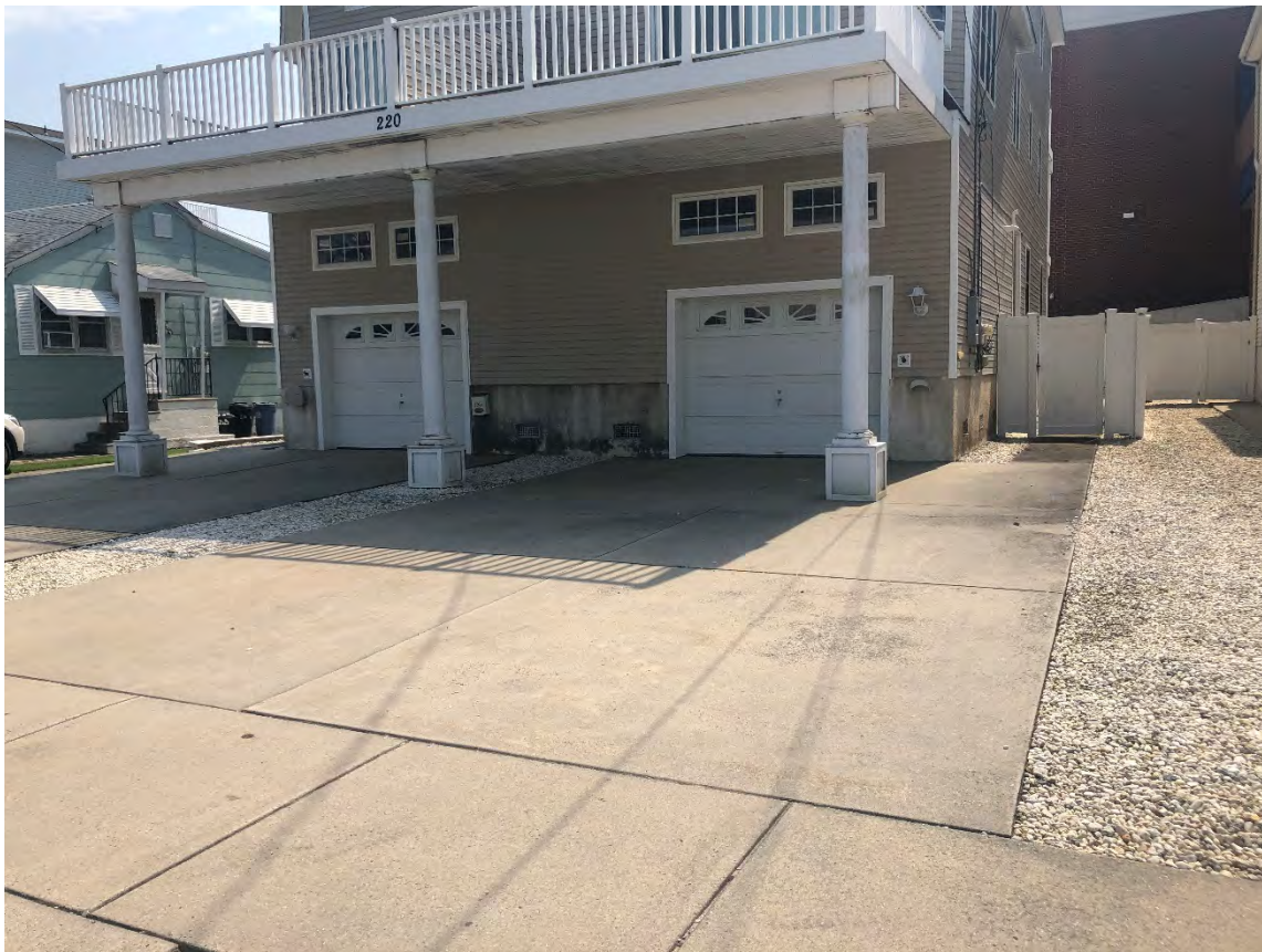
Photo No. 3 – West Front Exterior of 220 40 th Street
