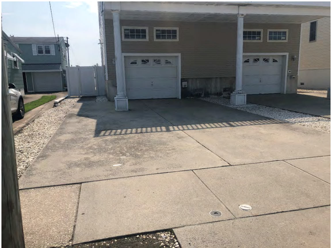
Photo No. 2 – East Front Exterior of 220 40 th Street
