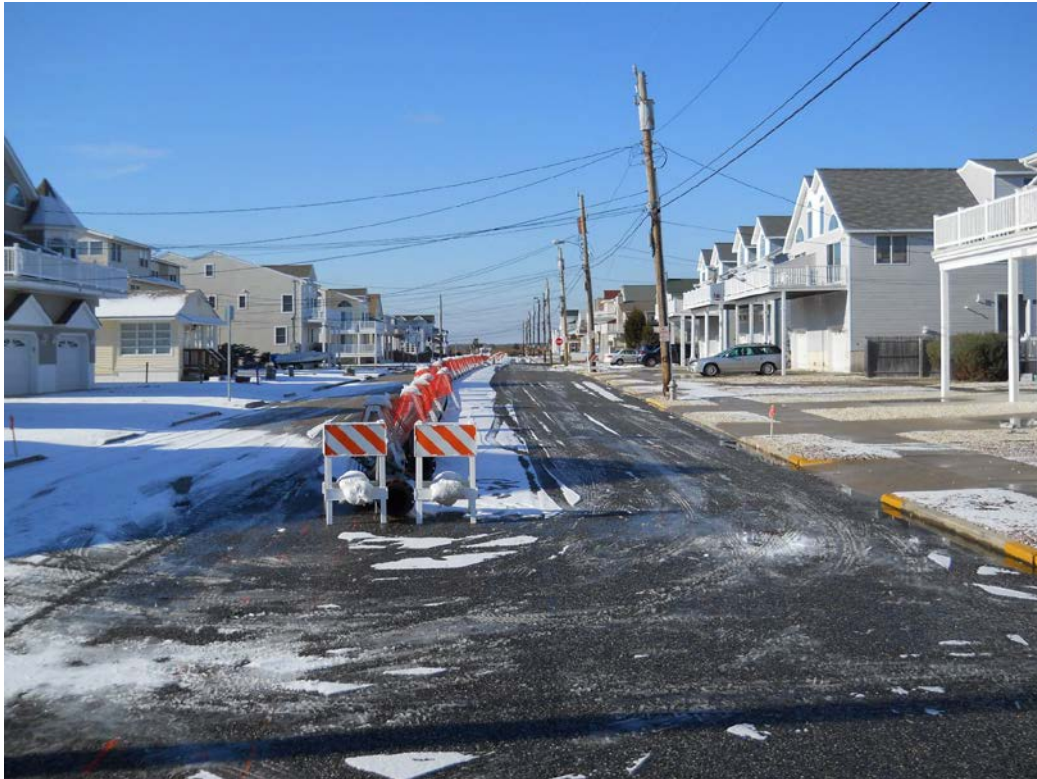
HDPE Piping for Depressurization System Running Along 39 th Street
