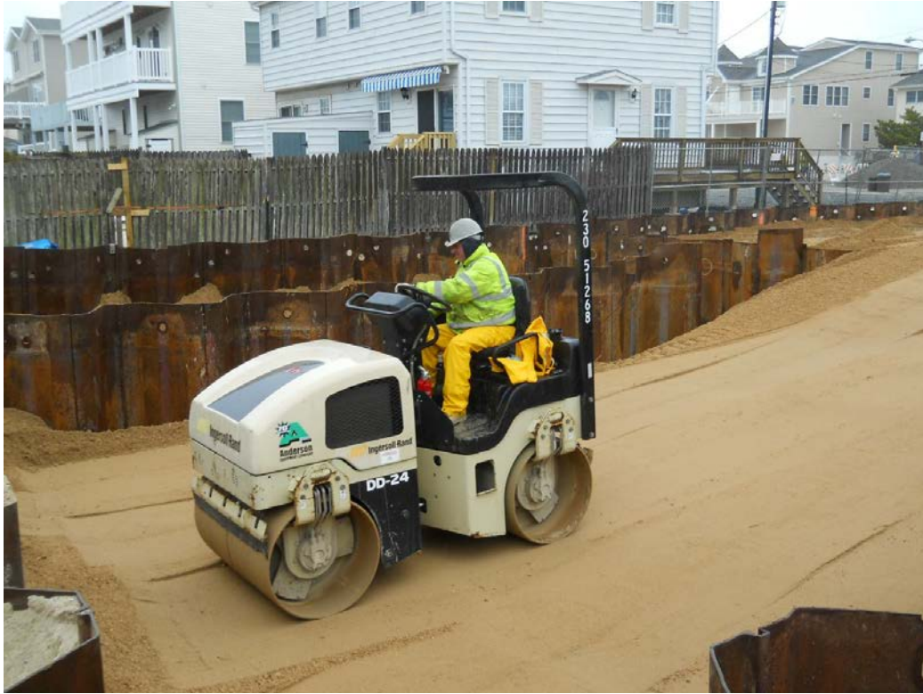
Compacting I5 material in Sampling Grid I2
