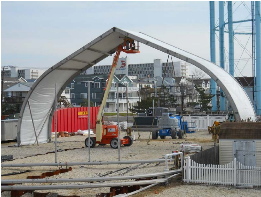
Constructing the Temporary Enclosure
