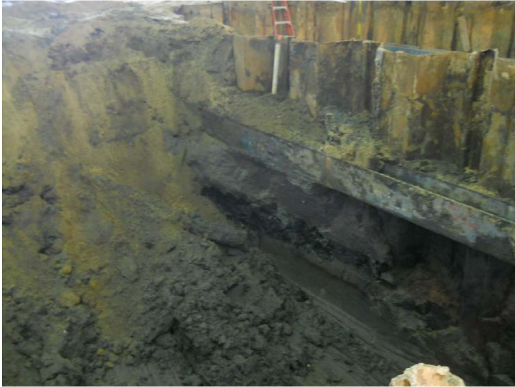
Excavating in Sampling Cell G2
