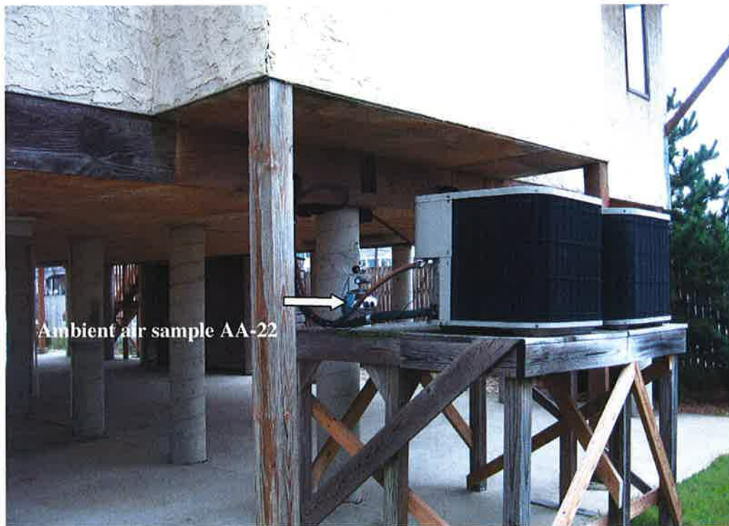
Photograph 11. 210 39 th Street: Location of ambient air sample AA-22 on the southwestern side of the vacant residential structure. The summa canister was placed on the platform approximately 5 feet off the ground.
