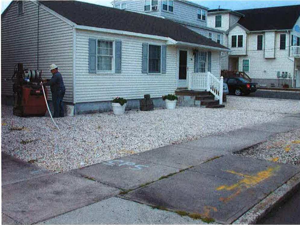
Photograph 1. 214 39 th Street: Temporary well point installation (TPZ-1).
