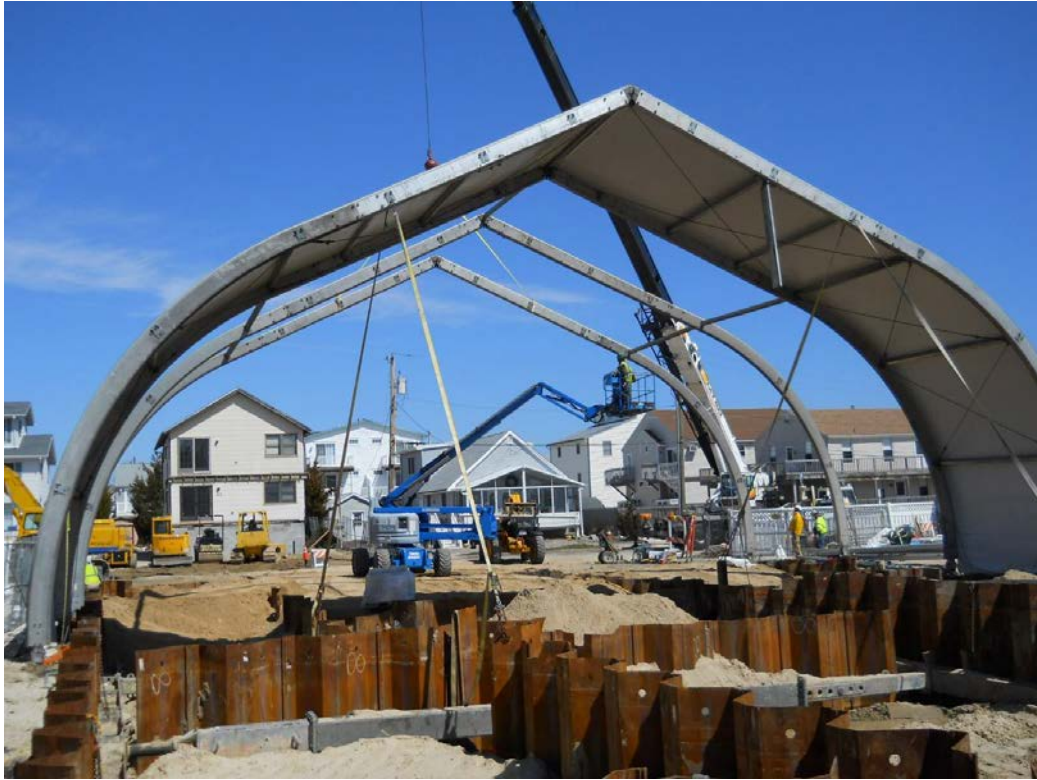
Disassembly of Temporary Enclosure
