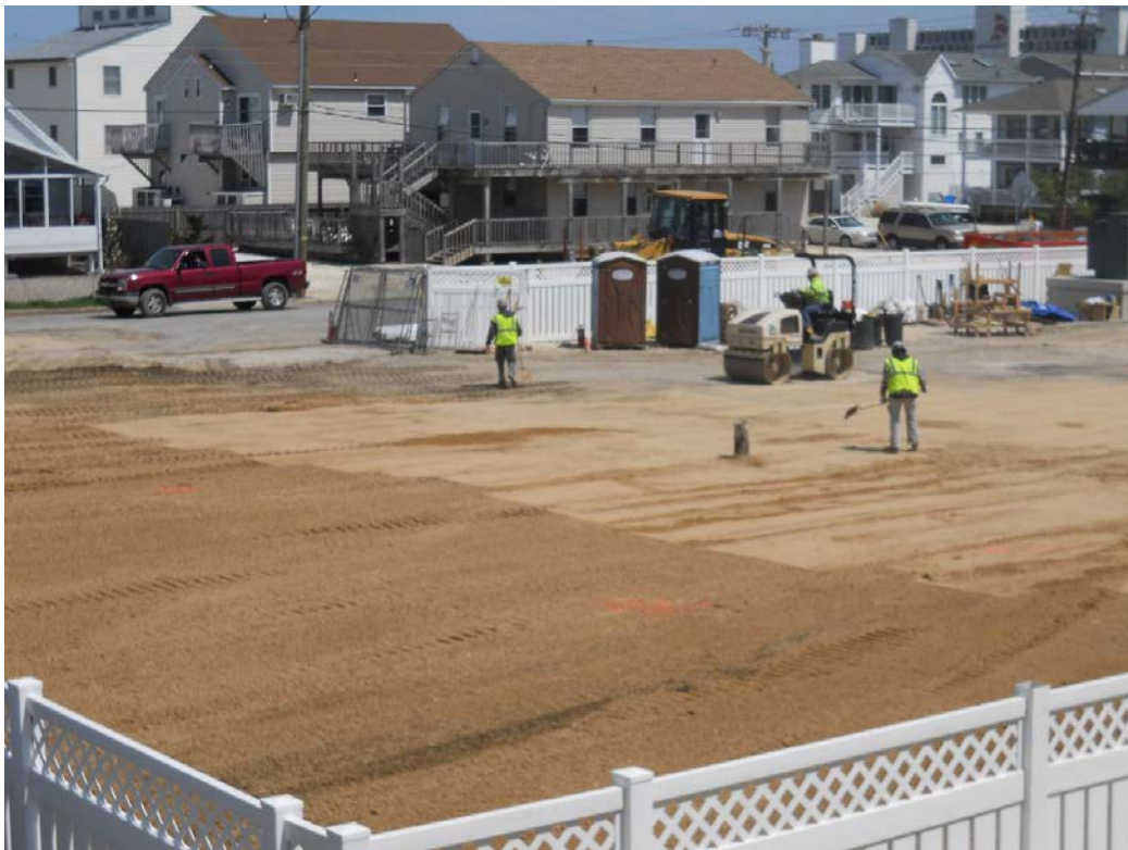
Compacting Fill Material at Final Grade Over the Work Area
