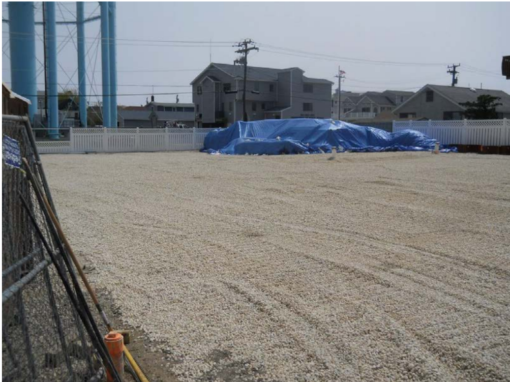
View of Site Looking East Showing Location of Stockpiled Sheet Piles
