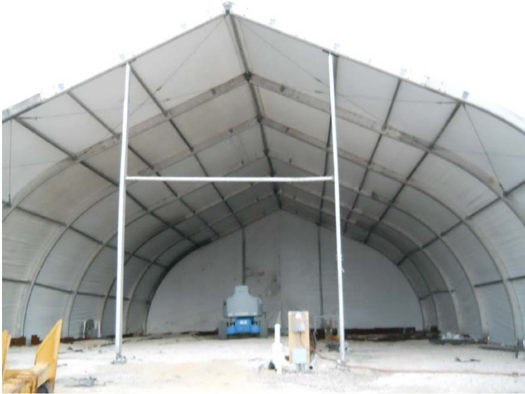
Interior of Temporary Enclosure
