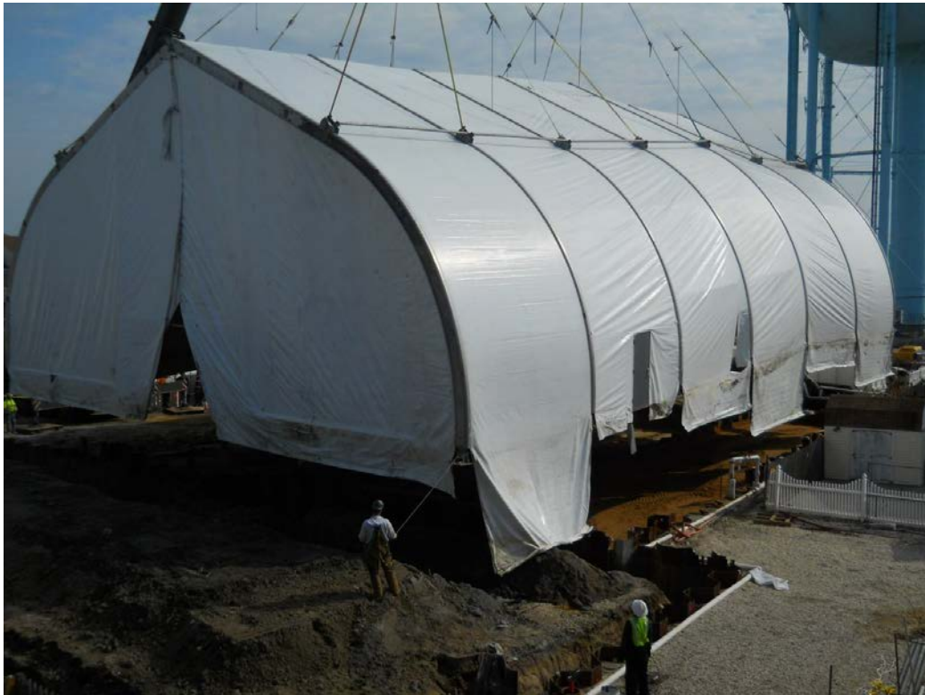
Moving Enclosure to Former 214 39 th Street Property
