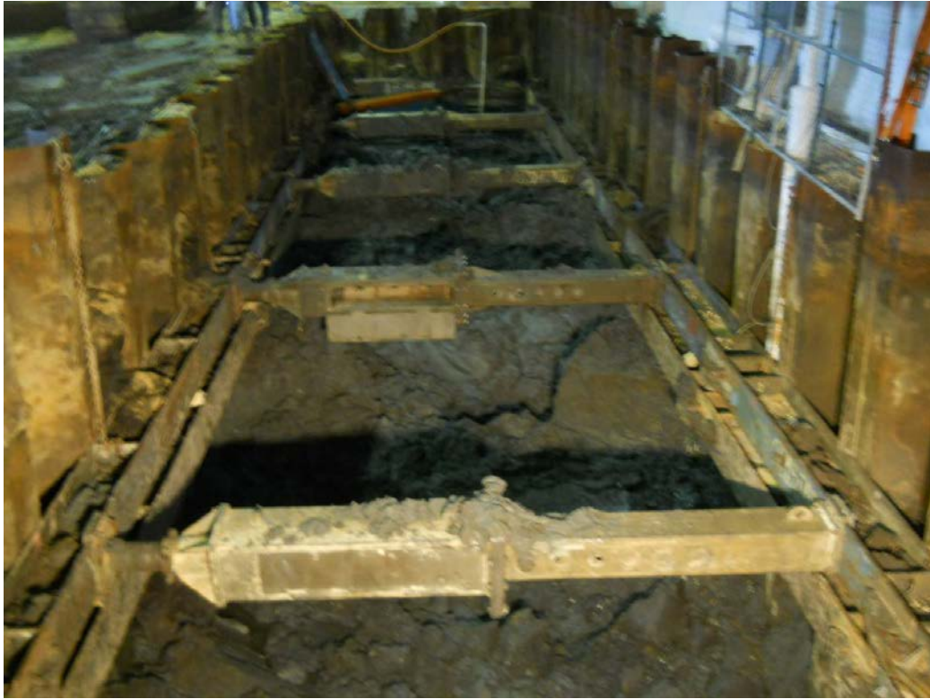
Interior Bracing in Sampling Grids I3 and I4
