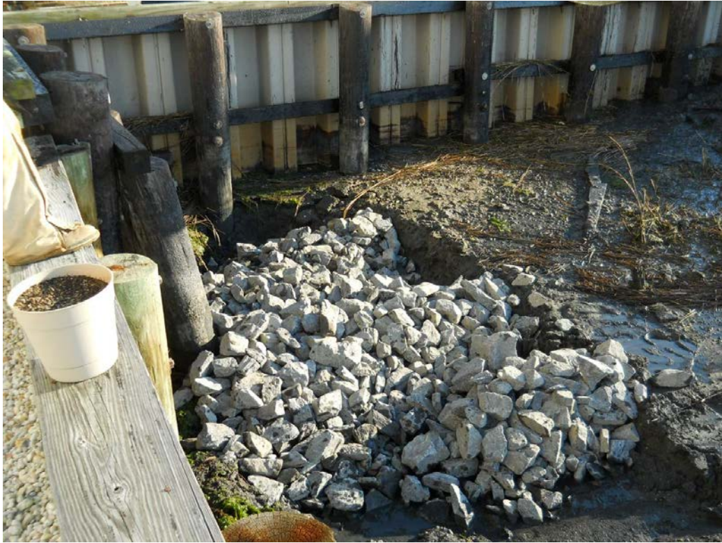
Energy Dissipating Rip-Rap Placed at 38 th Street Outfall
