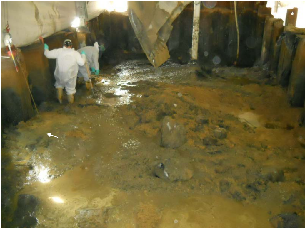
Excavating in Sample Grid G3
