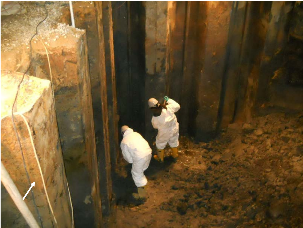
Hand Digging in I6 Below the Former Holder Base
