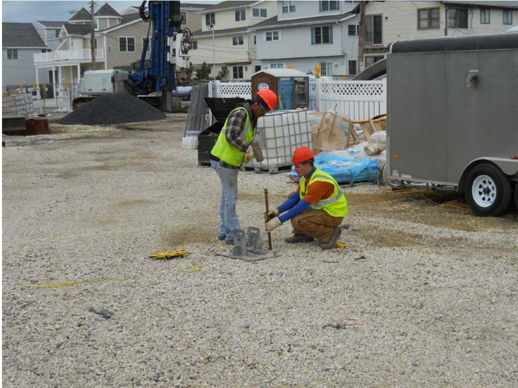
Setting Anchors for Temporary Enclosure
