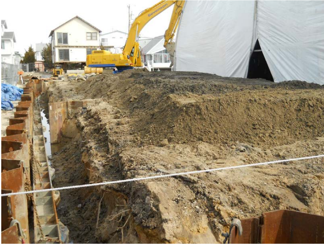
Former 214 39 th Street Property with Whalers Set Prior to Moving the Enclosure
