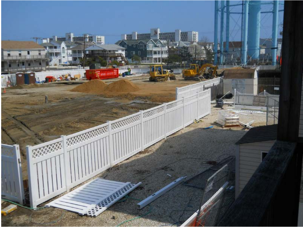
Installation of Perimeter Fencing
