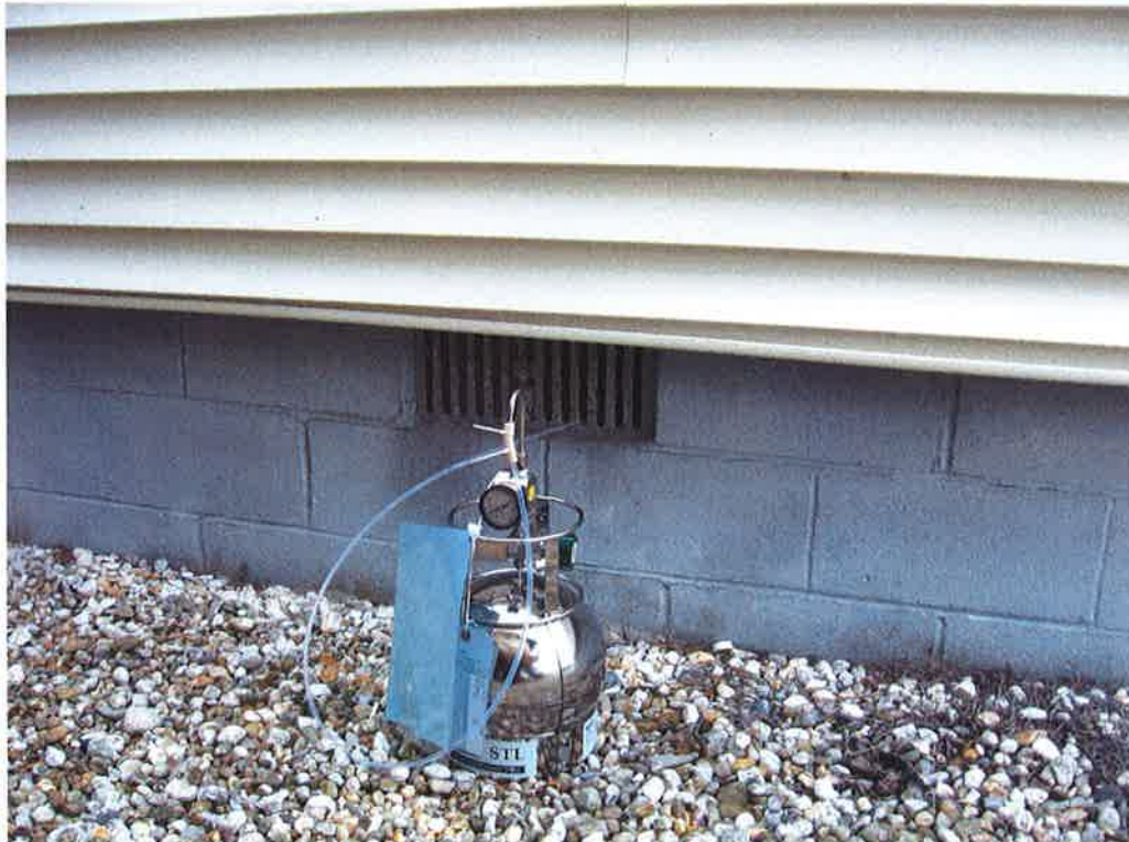
Photograph 10. 214 39 th Street: Crawl space air sample CS-34 collected through vent on the southeastern side of the residential structure.
