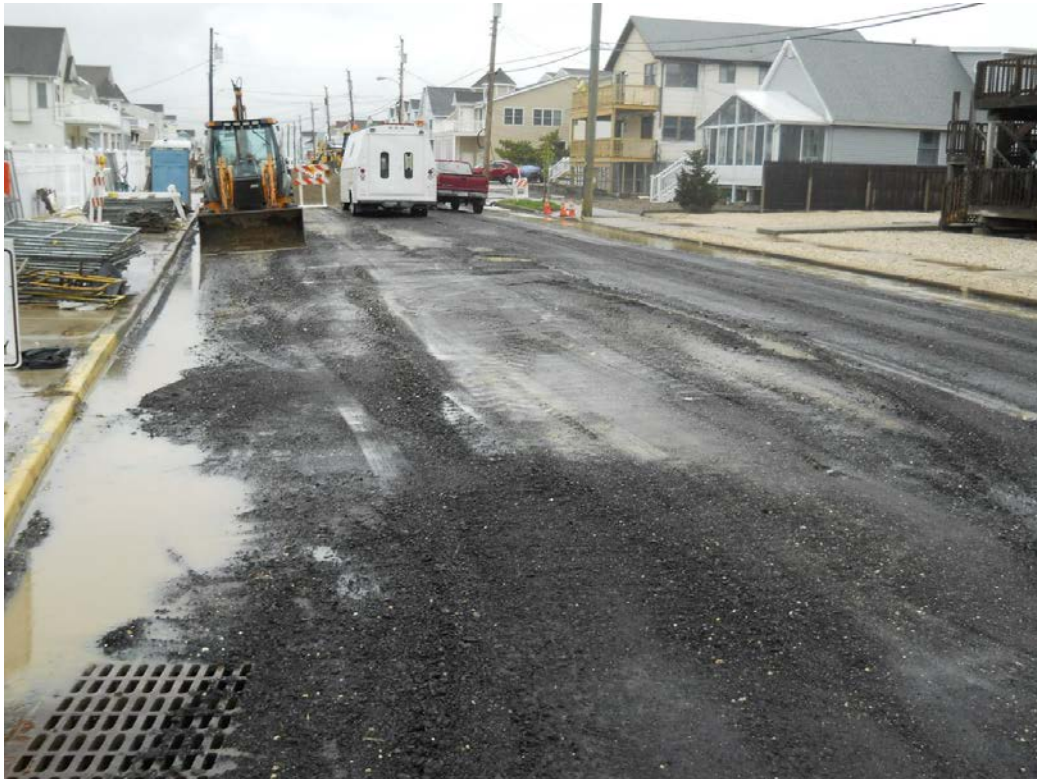
Completing Milling of 39 th Street
