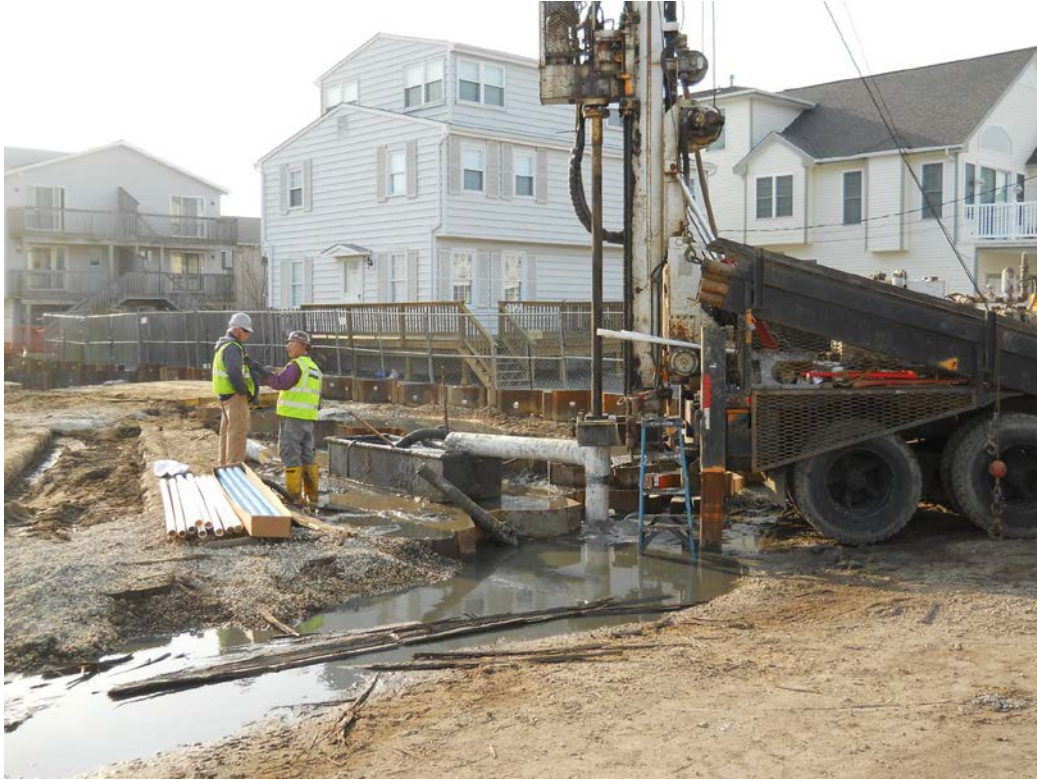
Installation of Inclinometer I9
