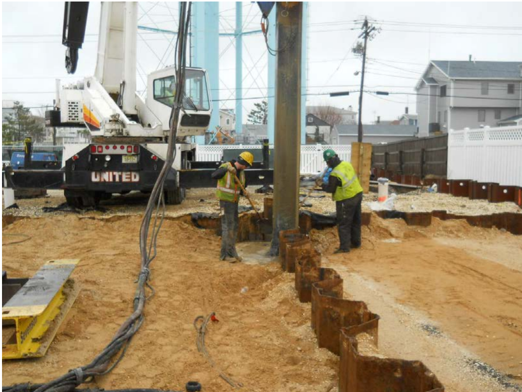
Removal of Interior Sheeting
