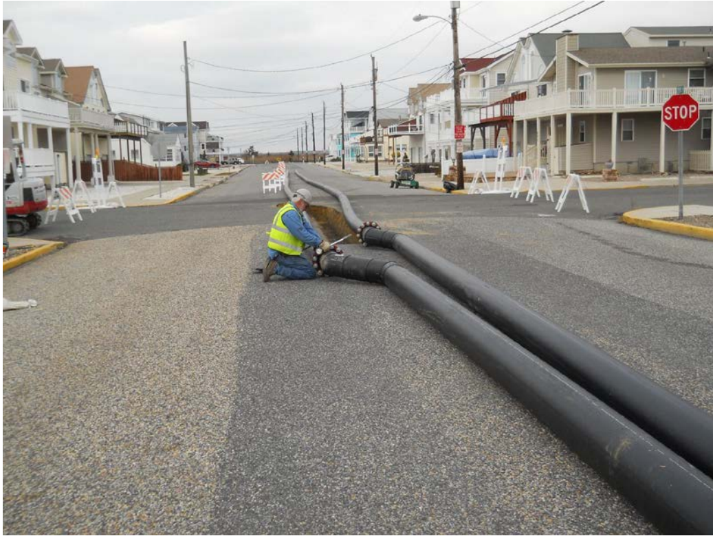
Installation of Road Crossings for Depressurization System Discharge Piping
