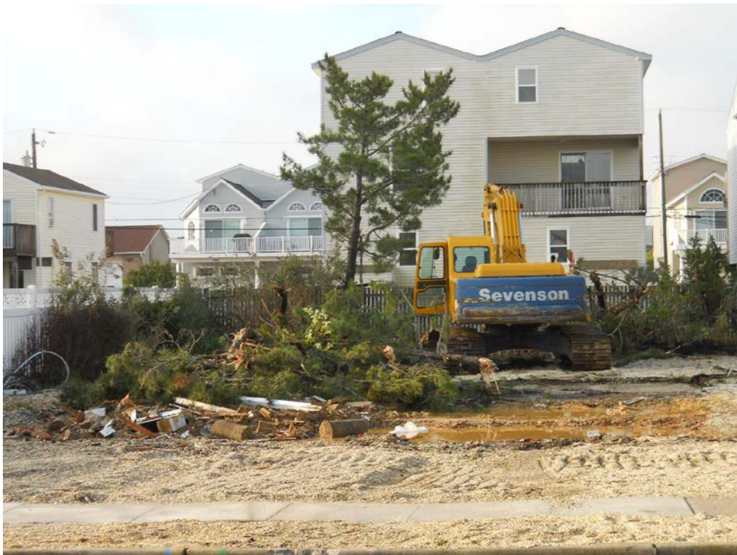
214 39 th Street Property after Building Demolition
