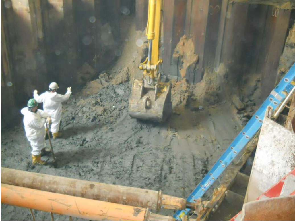
Excavating in Cell I2
