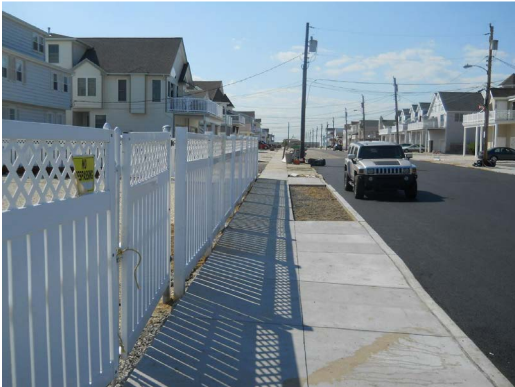
Completed Sidewalk and 39 th Street Repaving
