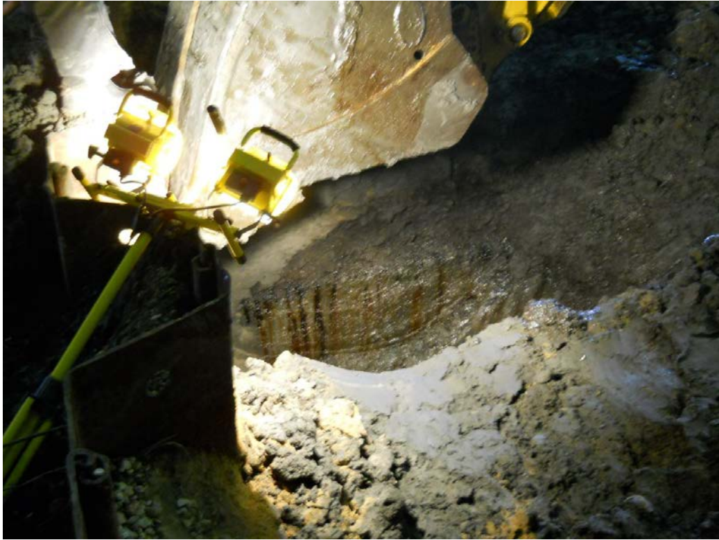
MGP Impacts Visible During Excavation Activities in I5
