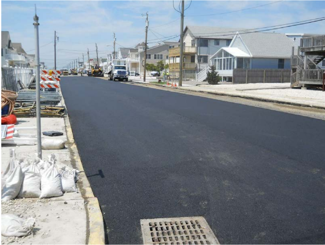
Repaving 39 th Street
