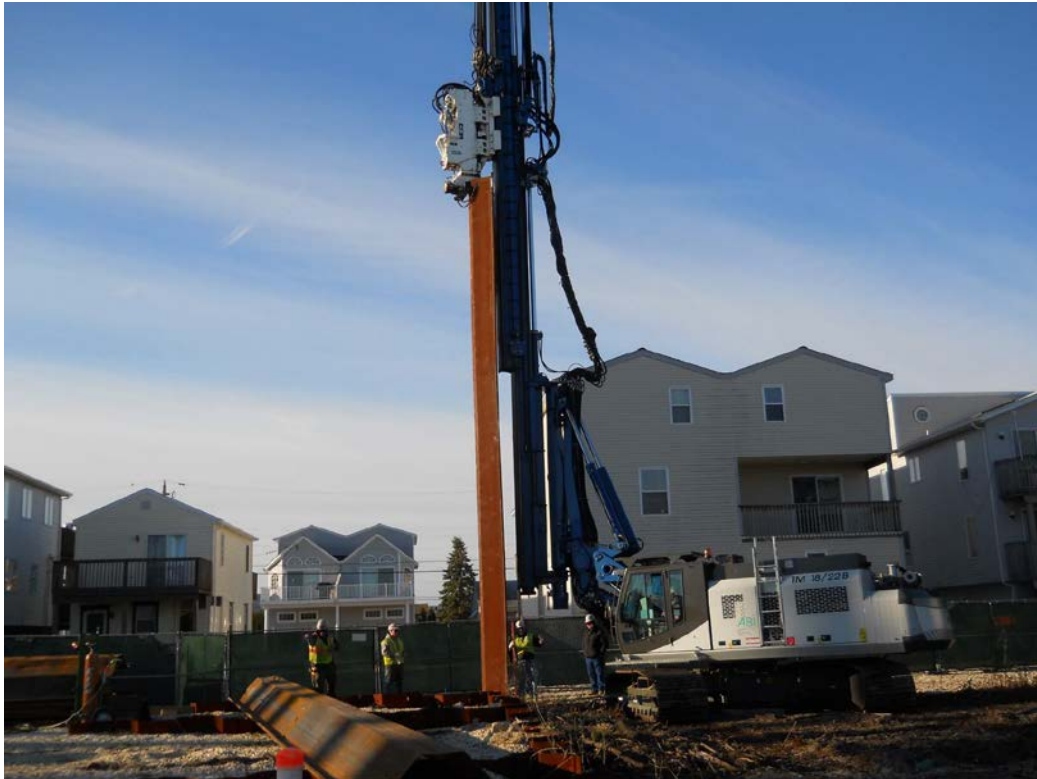
Advancing Sheet Piles at Former 214 39 th Street Property
