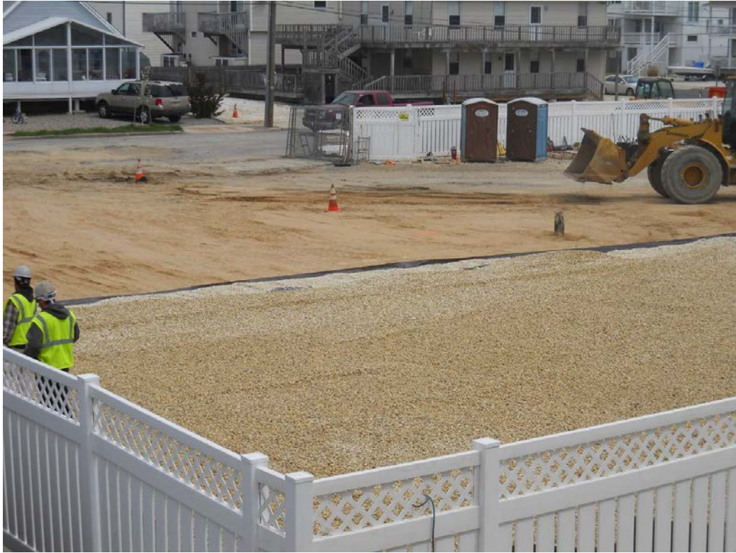
Placement of Stone and Geotextile over site
