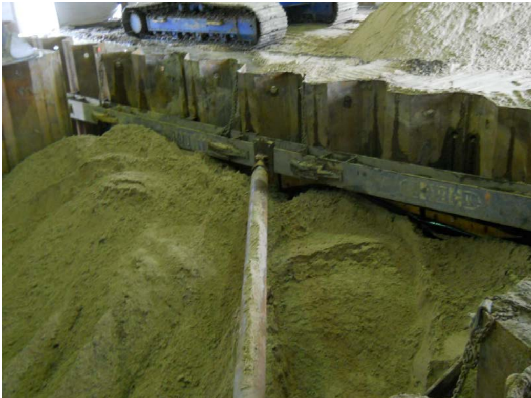
Backfilling in Sampling Grids F1 and G1
