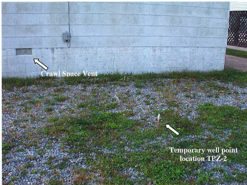
Photograph 4. 205 40 th Street: Installed temporary well point TPZ-2 in relation to the crawl space vent on the northeastern side of the residential structure.
