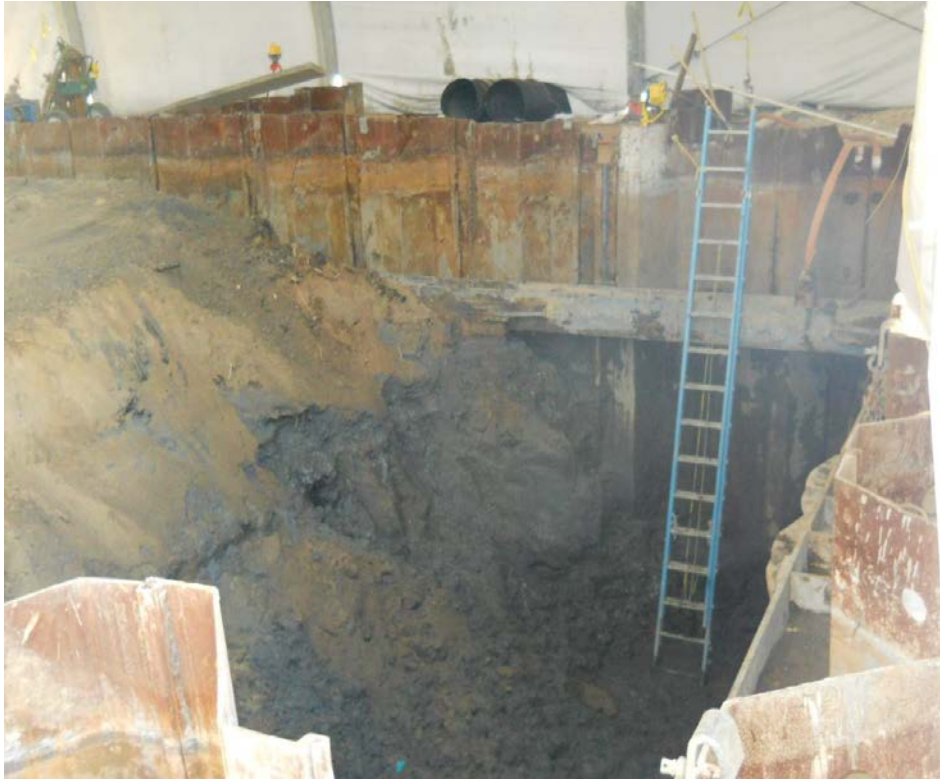
Excavating in Sampling Cell I1
