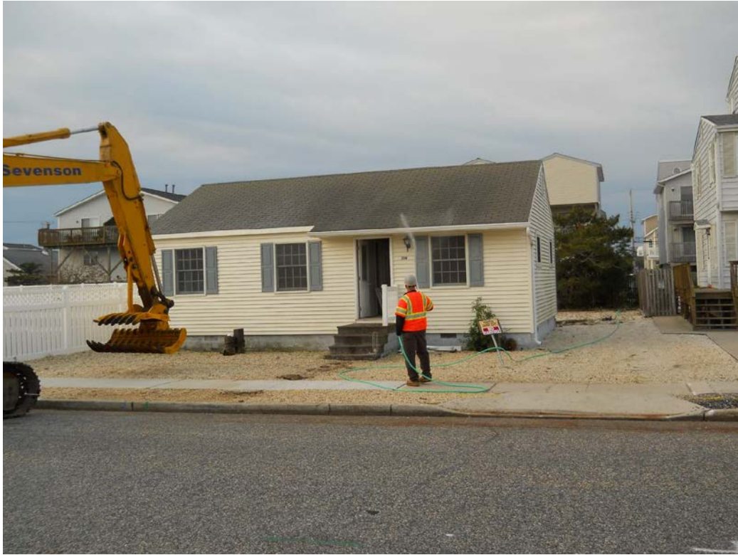
214 39 th Street Prior to Demolition
