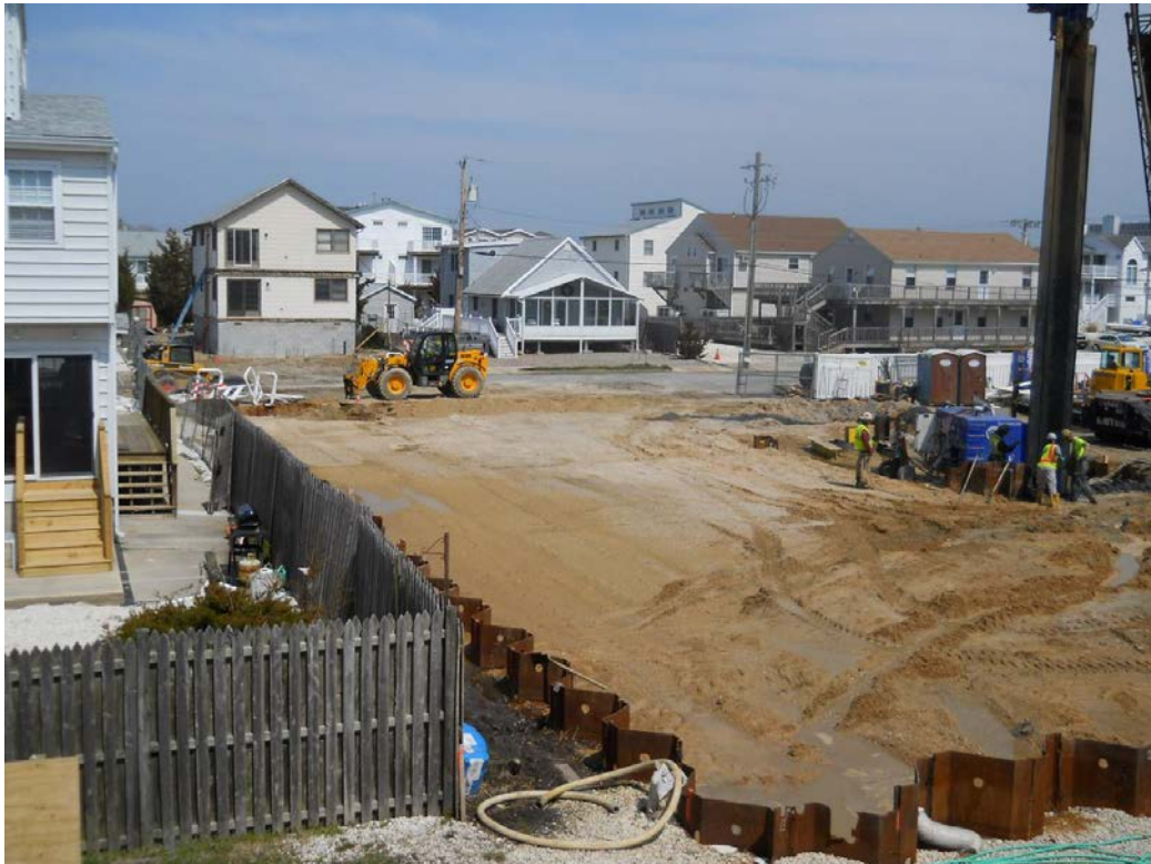
Former 214 39 th Street Property after Final Backfill Grading
