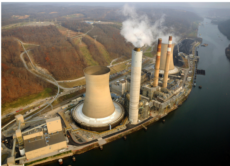
Fort Martin Power Station is located in Madsville, West Virginia, along the Monongahela River.
