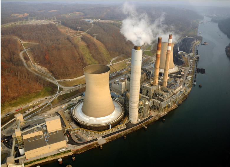
Fort Martin Power Station is located in Madsville, West Virginia, along the Monongahela River.
