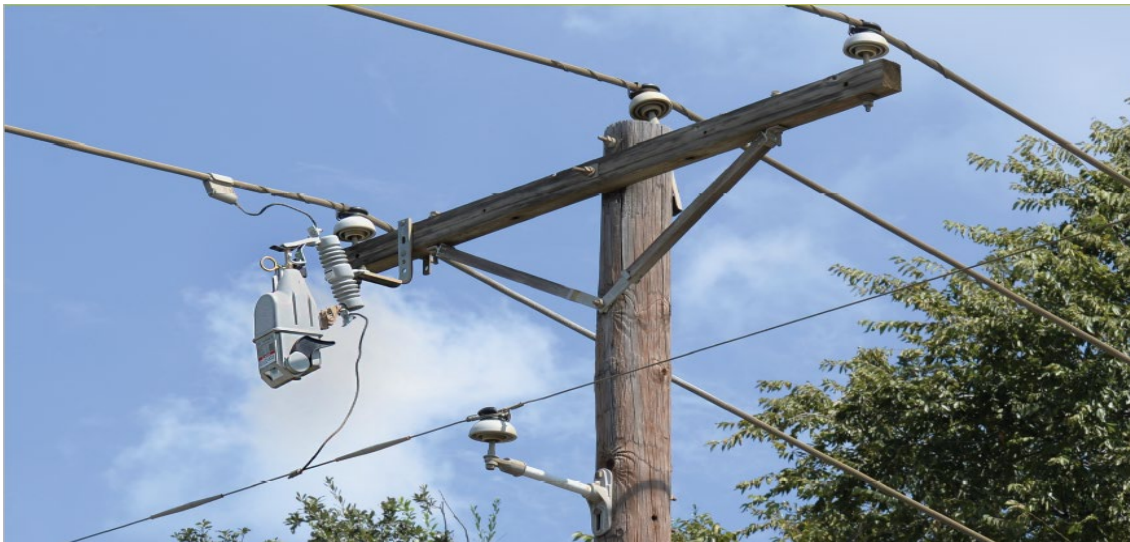
Figure 13: TripSaver II – Field Installed Device
