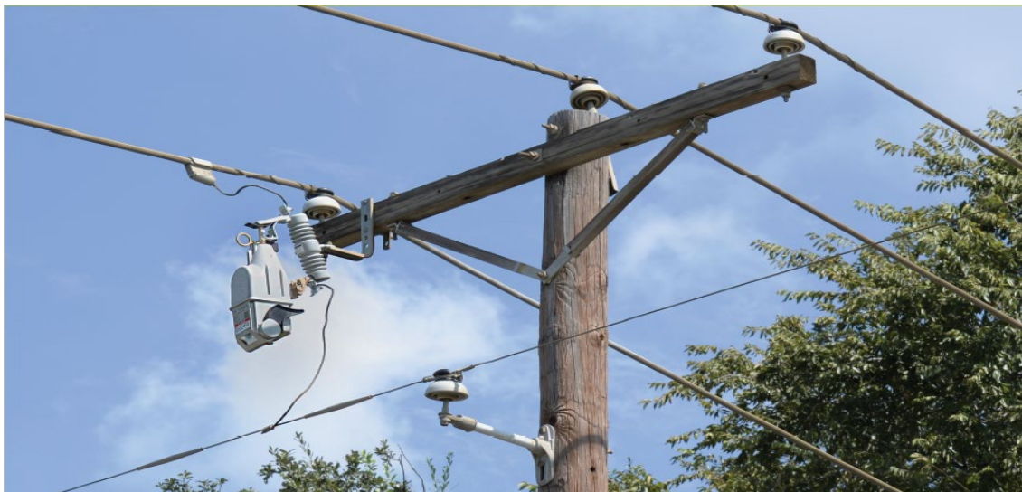
Figure 13: TripSaver II – Field Installed Device
